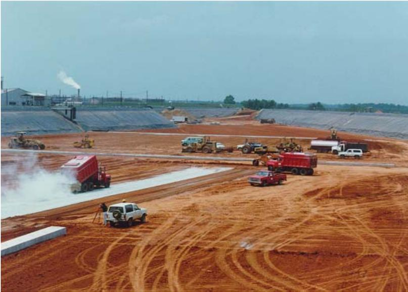
Lining waste water lagoons or landfills with smectite to prevent toxins from leaking through and contaminating the ground water.
